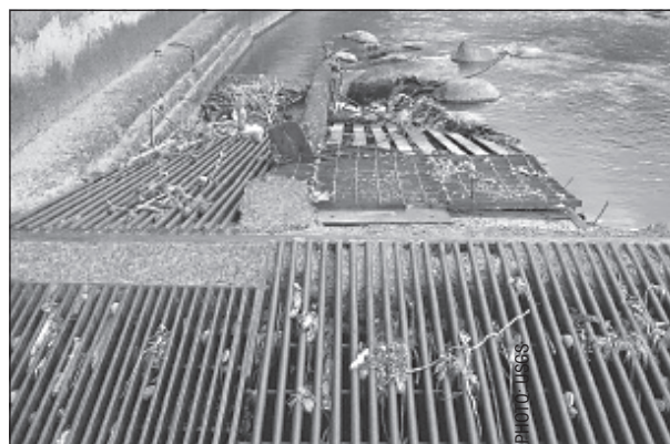
Spreckels Ditch diversion intake on south side of 'Iao Stream. Closeup of parts of intake grate, June 6, 2006.
